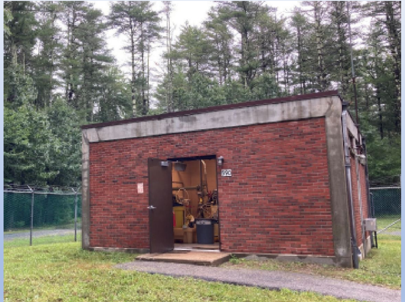
Mayflower Well No, 1 Pumping Station
