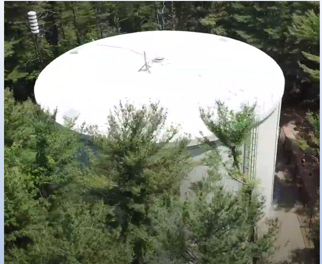
Captain's Hill Water Tank
